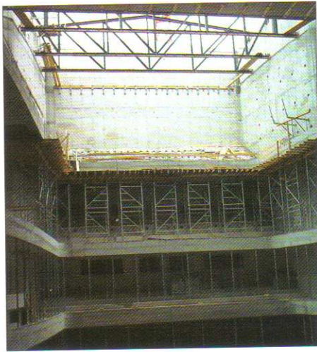
Fig. 2: Rear of the auditorium during construction
