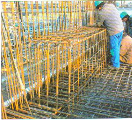
Fig. 5: Reinforcement of upstanding lug
