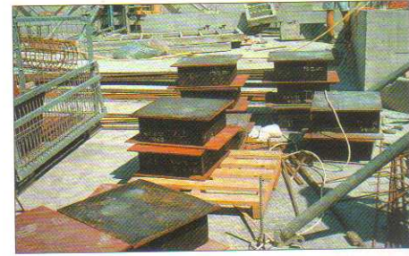
Fig. 4: Natural rubber bearings on the site
