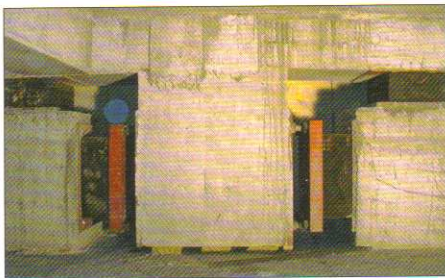
Fig. 6: Lateral bearings between lugs
